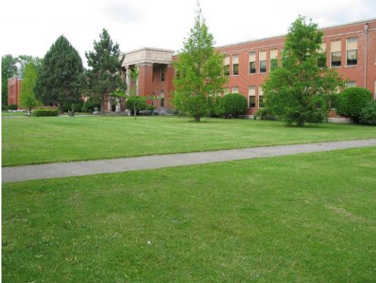
East elevation of main building (217A).
