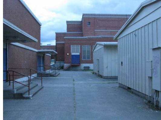
View of area near auditorium (217E), portables (217P1 and P2), and new gymnasium (217J).
