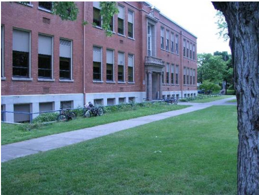
South side of south wing (217D).
