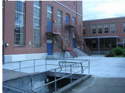
Auditorium (217E) and entrance into subsurface cafeteria, looking east.
