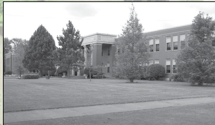
2009 photograph of main entry (East elevation).
